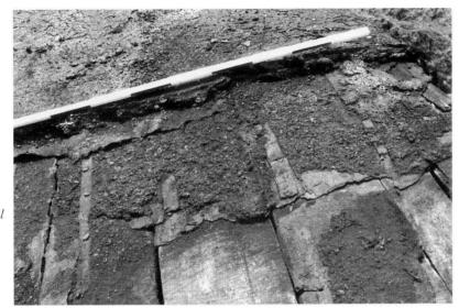
Fig. 17 Paisley House, Oxford Detail of roof showing boards, paper, card fixing strips and composition coat. Oxford Archaeological Unit
